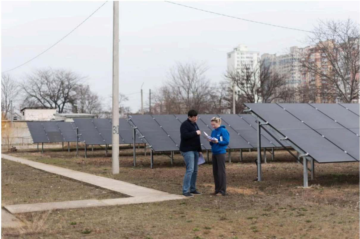
Solar panels to power water pumps during blackouts.
